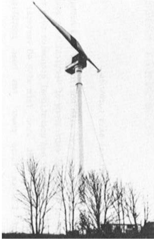
Fig. 5: Single blade with counterweight wind rotor design.
